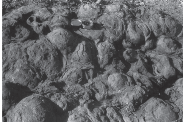
Fig.6.4 : Exfoliation (Flacking) and granular disintegration
