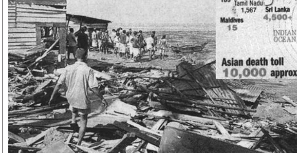
People walk through debris of their houses destroyed by tidal waves on the coastal area in Colombo, Sri Lanka
