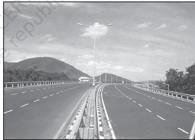
Fig. 8.3 : Dharmavaram Tuni National Highway, India
