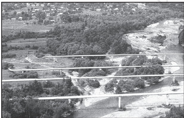
Fig. 8.17: Pipelines transporting natural gas in Ukraine
