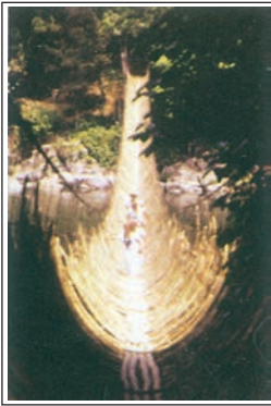
Figure 6.7 : Rope Bridge (Arunachal Pradesh)
