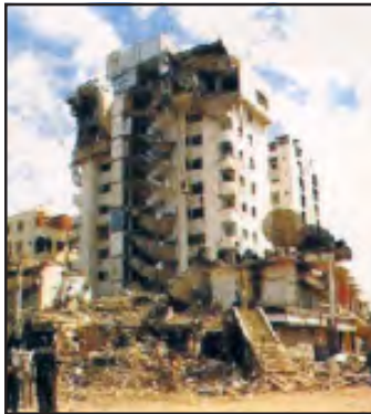
Fig. 3.3a: Destruction caused by an Earthquake in Gujarat
