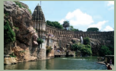
Fig. 4b. Chittorgarh Fort, Rajasthan
