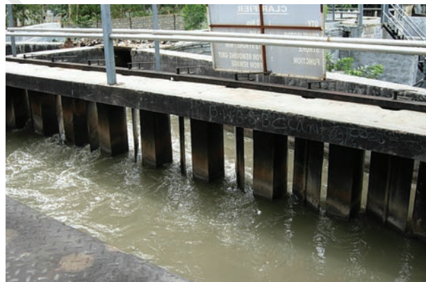
Fig. 18.4 Grit and sand removal tank
