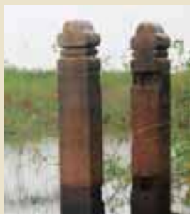
Piston sluice installed during the Pandya period in Pudukkottai Region
